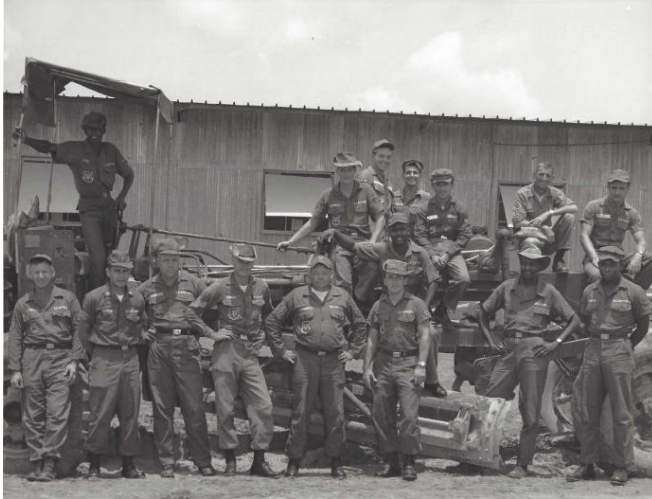
Electrical Crew (Sorry cannot remember individual names)
