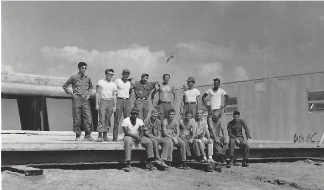
SSgt Ebbert and the Da Nang Marine Evacuation Hospital Erection Crew
